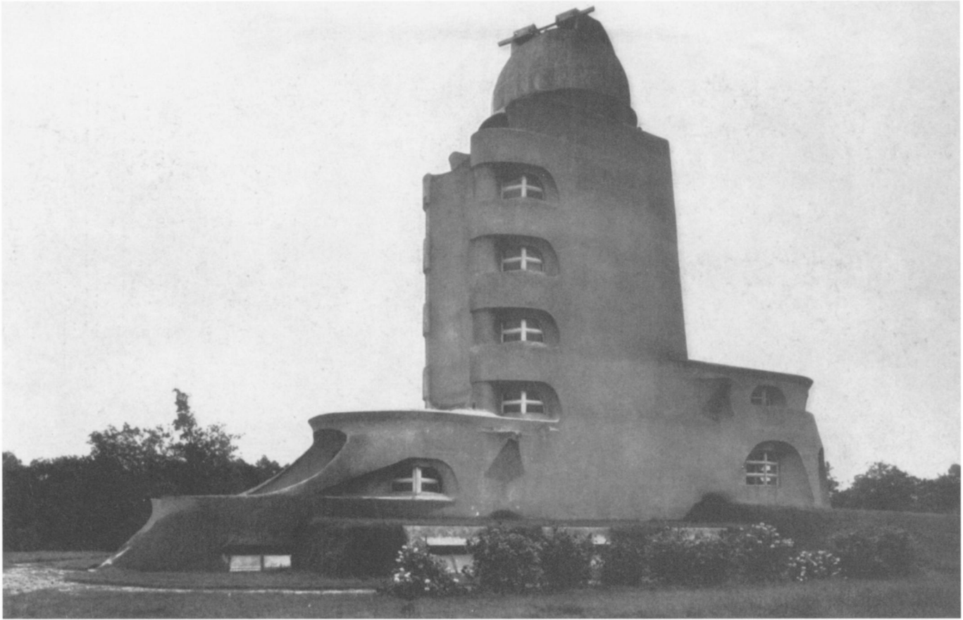
FIG. 1: Erich Mendelsohn, Einstein Tower, Potsdam, Germany. Designed 1917–20, constructed 1920–21. Note the grass-covered platform of the underground laboratory.
