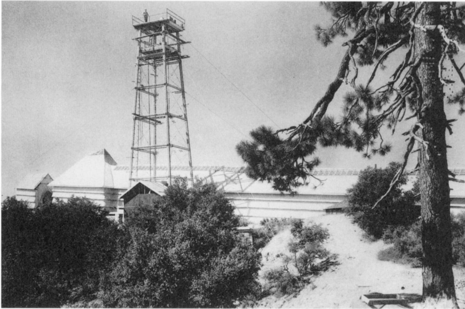
FIG. 10: Vertical coelostat and horizontal laboratory, Snow Telescope, Mt. Wilson, Pasadena, California, 1907. The coelostat tower was the second built on the site.
